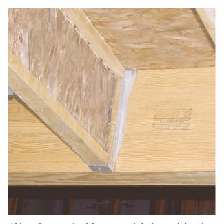
Although recognized for exposed designs, glulam is a workhorse in hidden framing, as well.
