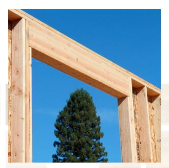
Glulam beams make strong, stable headers for framing window and door openings.
