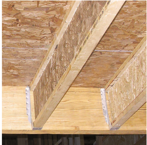
Glulam in I-joist compatible depths is commonly used in residential floor framing.
