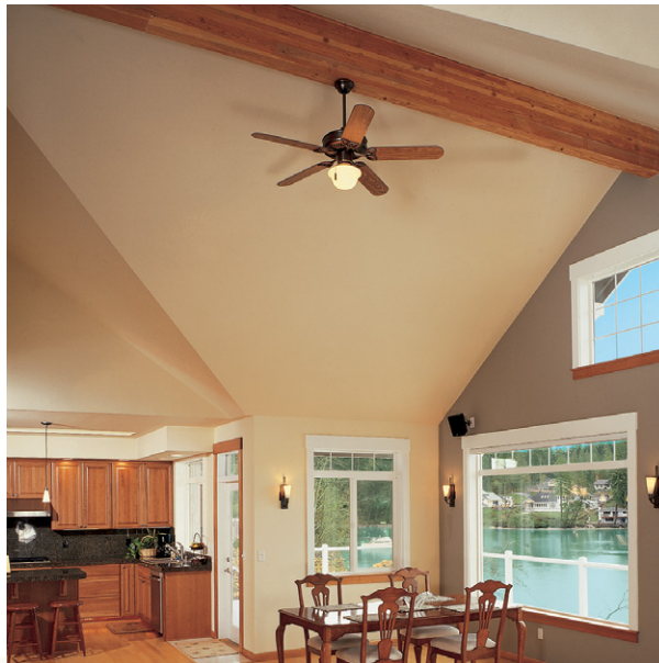
Glulam ridge beams are ideal for the dramatic roof lines and open spans popular in today's home.
