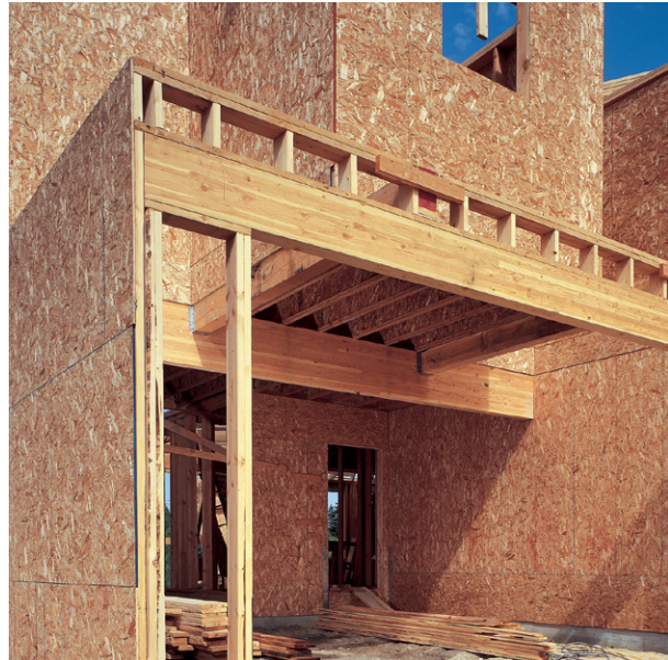
Glulam garage door header extends over adjacent narrow shear wall.
