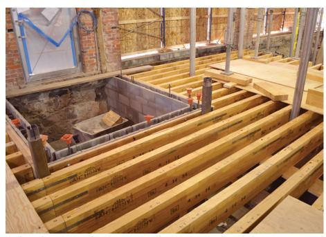
The floor is framed with 20-foot, 3-1/2-inch-by-9-1/2-inch glulam beams spaced 12 inches on center.
