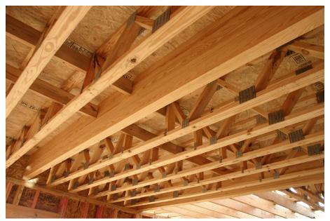
Glulam beams combined with trusses create an open, flexible floor plan.
