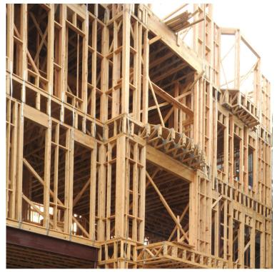
Glulam beams span the full width of the rowhouses' floor systems, helping to eliminate interior load-bearing walls, and were also used for window headers and some garage door headers.
