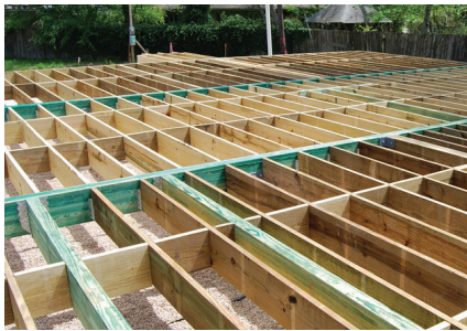
Raised Floor Construction
