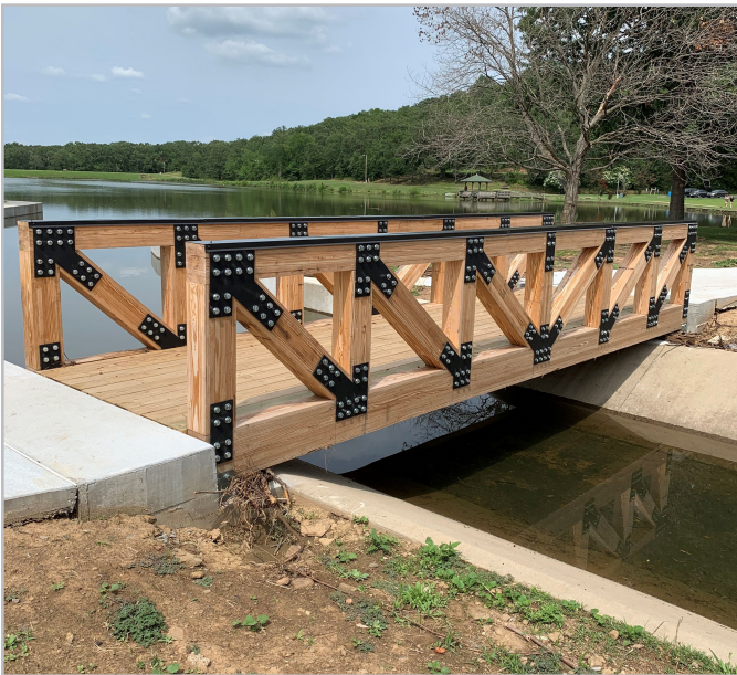
Power Preserved Glulam® Bridge Application
