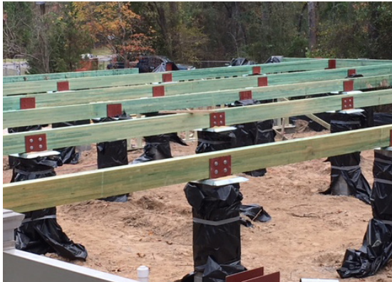
Power Preserved Glulam® Pier and Beam Application
